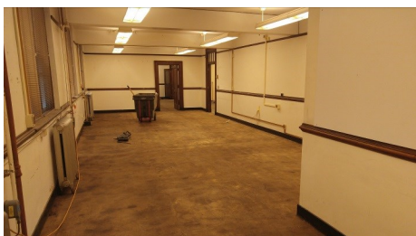
A view of the Admin Office in May 2017.
