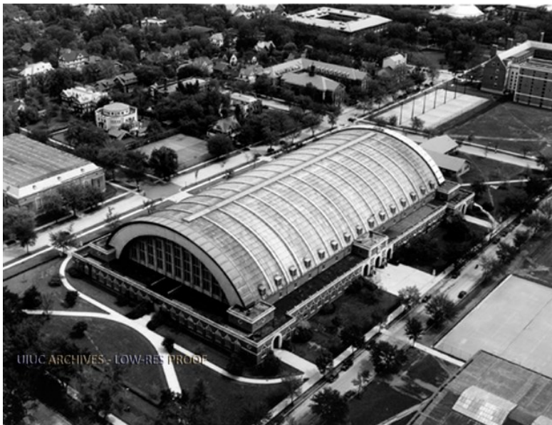
An aerial view of the Armory Building, photographed on 13 May 1935.
